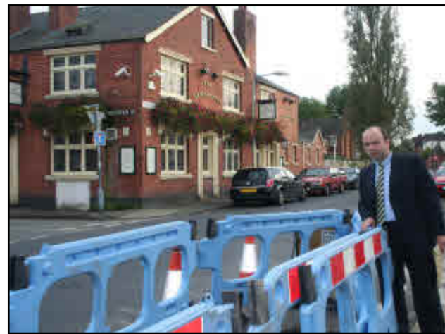
Cllr Robin Lawrence checks out the Riches Street work
